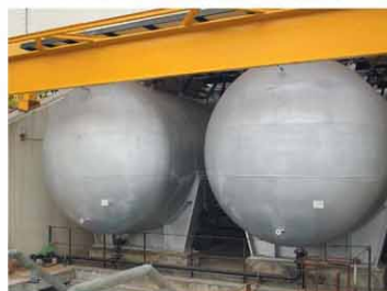
Surge Vessel (11M x 4.5M) 壓力緩衝儲缸製造
